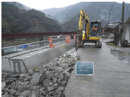
(既設舗装版撤去)
