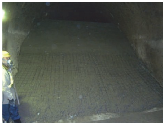
(溶接金網設置)
