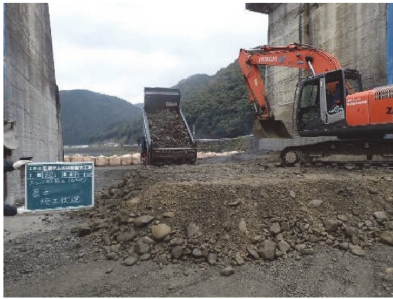
(土砂敷設状況)
